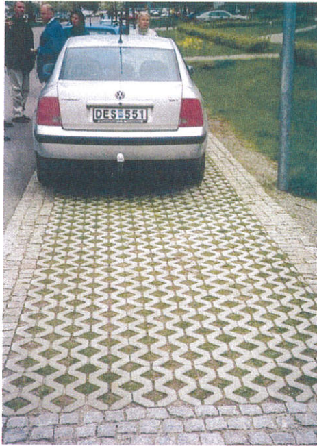
Figur 6. Markarmering betonghålsplattor.
